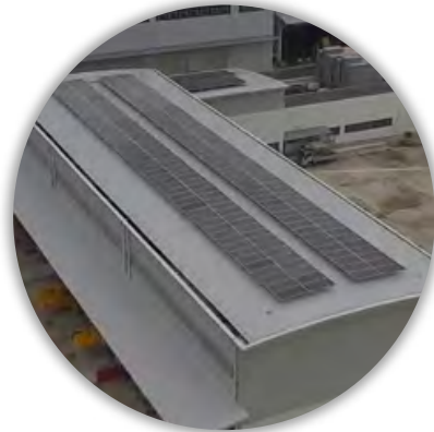
Solar Panel Systems
