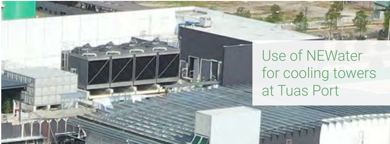
Cooling Towers at Maintenance Base, Tuas Port
