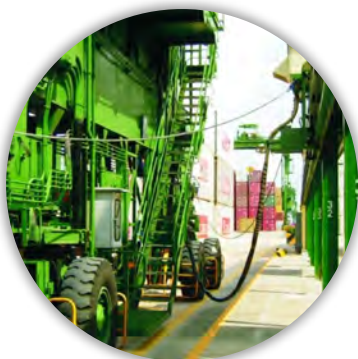
Electric Rubber Tyre Gantry Cranes
