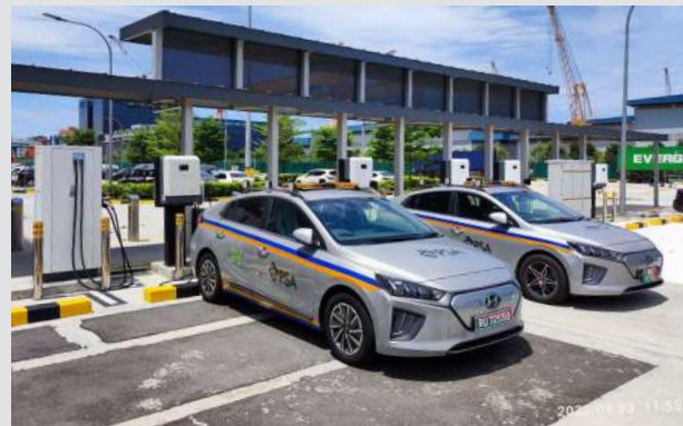
Electric vehicles charging infrastructure at Tuas Port
